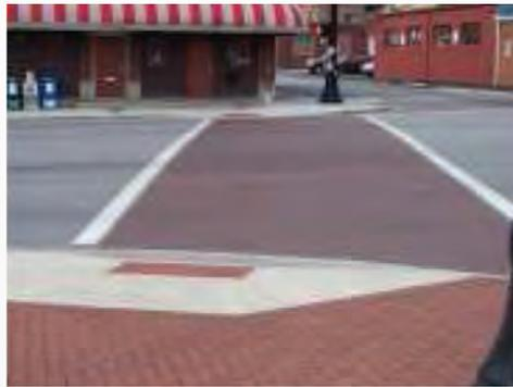
*Figure 56: Detectable Warning Surfaces*
