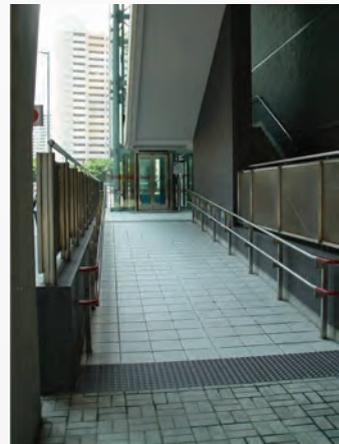
Figure 203: Dual Height Handrails
