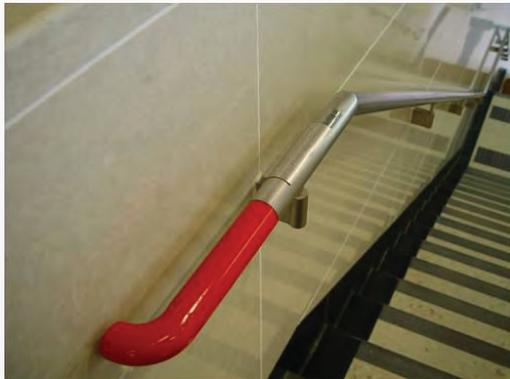
Figure 202: Handrail Extensions
