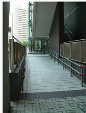
Figure 203: Dual Height Handrails
