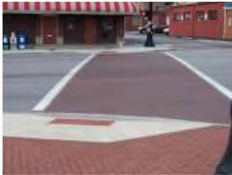
*Figure 56: Detectable Warning Surfaces*
