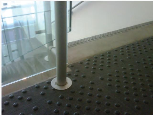
*Figure 216: Detectable Warning Surface at Top of Stair*
