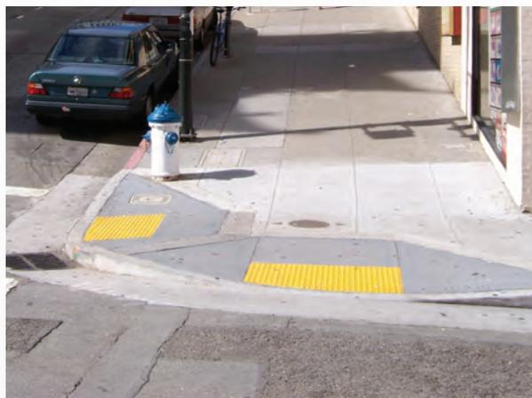
*Figure 215: Detectable Warning Surface at Kerb cut*
