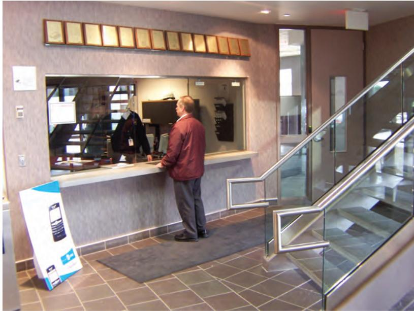
Figure 176: Detectable Handrail
