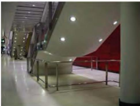
*Figure 38: Detectable Barrier*
