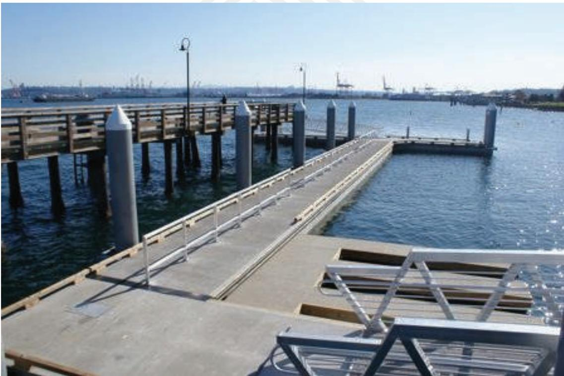
*Figure 90. This illustration indicates some of the features that may contribute to creating access: almost level through-surfaces, ramped access across different heights, railings to designate ends of platforms and flexible junctions.*
