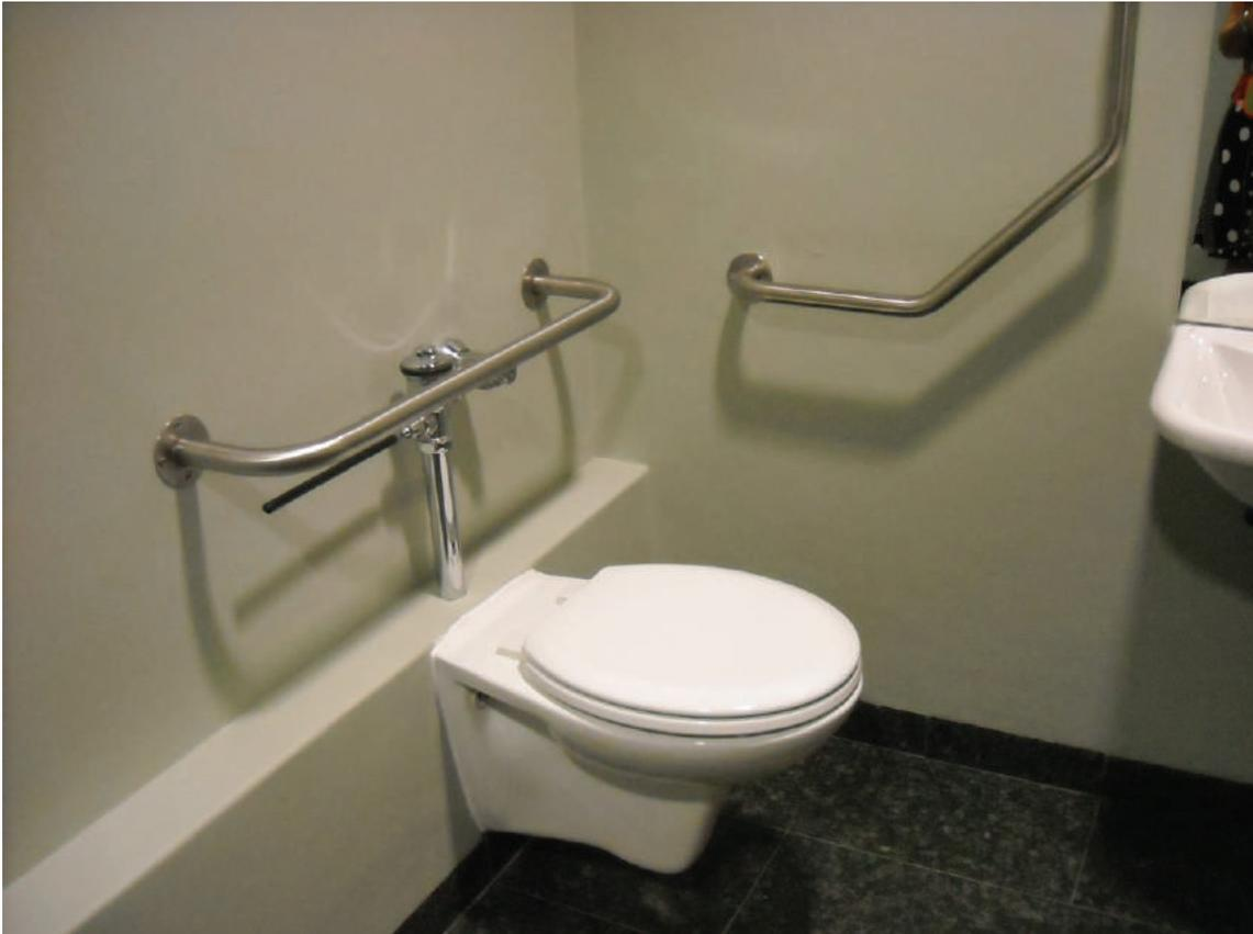
Figure 26. An illustration of the typical placement of the components within an accessible toilet configuration.
