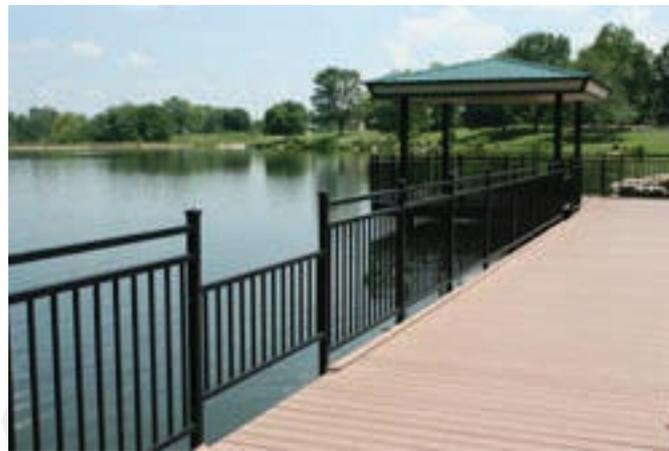
*Figure 94. An example of a lowered portion of platform fencing for access by shorter users, children and seated users to fish.*
