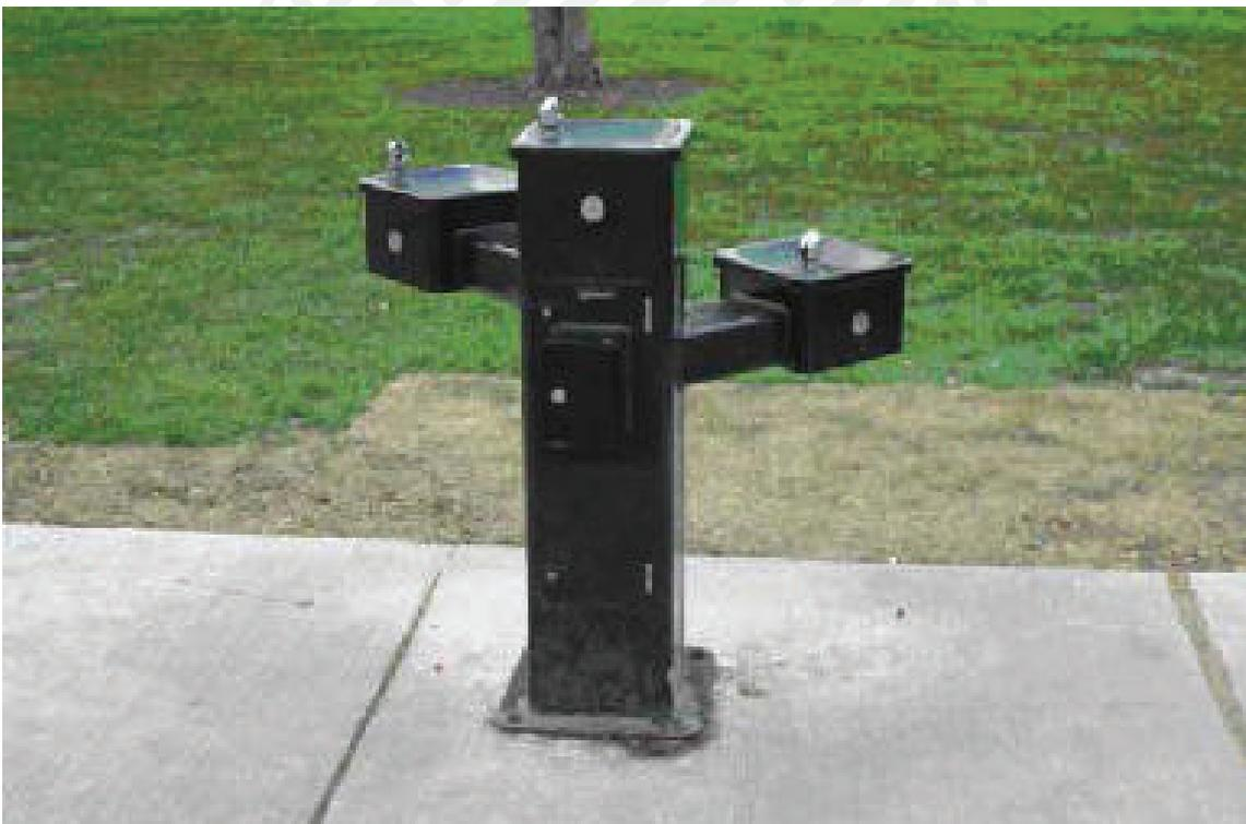
*Figure 71. Drinking fountains at multiple heights. Although useful, absolute best practice would be ensure that there is a vertical base from the spout to the floor.*
