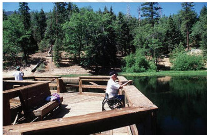
*Figure 95. An example of the manner in which lowering the entire portion of balustrading and edge-protection over water enables all users to be able to both view water-scapes, as well as to enjoy potential fishing experiences.*
