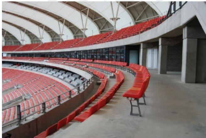
*Figure 96: This picture, taken in South Africa, prior to the 2010 World Cup, illustrates an example, in practice, of clear circulation space, located behind seating.*
