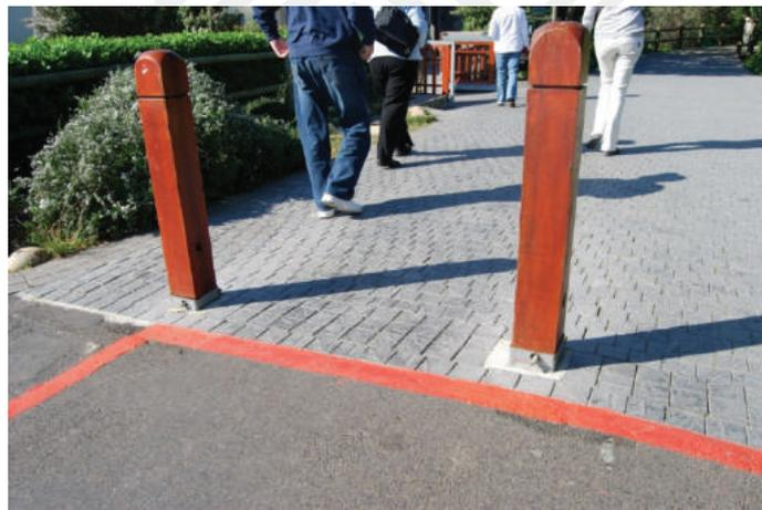
*Figure 89. Using color to demarcate spaces, as well as differences in floor surfaces to indicate different usages, contribute to the usability of environments. This is also a good example of how bollards can be employed to stop vehicular traffic, yet still retain the sufficient width to allow assistive mobility devices to gain access.*
